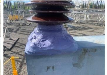
Build up Belzona product, ensuring no air pockets remain. Product given a week to cure before 5 bar restored to the Gas Circuit Breaker
