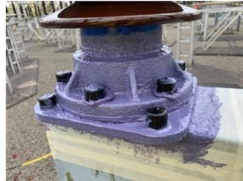
Cover nuts/bolts with belzona filled caps
