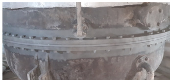
Surface preparation by grit blasting
