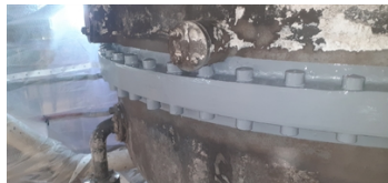
Finally full encapsulation of repairs using Belzona 5811
