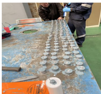
Application in progress of the nozzle inserts
