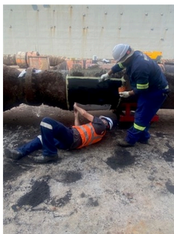
Hoses being prepared ready for Application in progress repair
