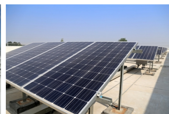
Solar panels fitted
