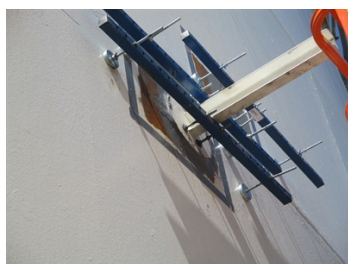
Brackets being bonded in place
