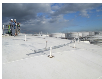
Brackets bonded in place
