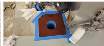
Second drain, application with Belzona 4311
