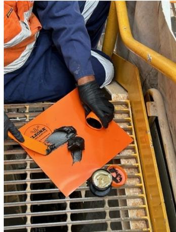
Mixing Belzona 1212 in preparation for the repair
