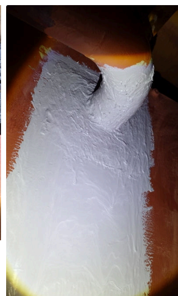
Surface coated with Belzona 1391T
