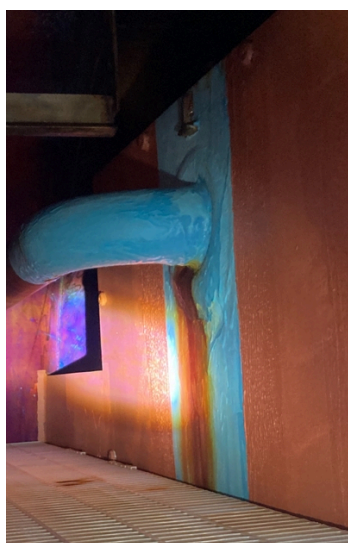
Before the surface preparation
