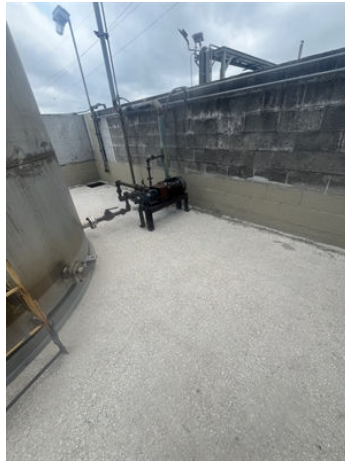
Area after grit blasting
