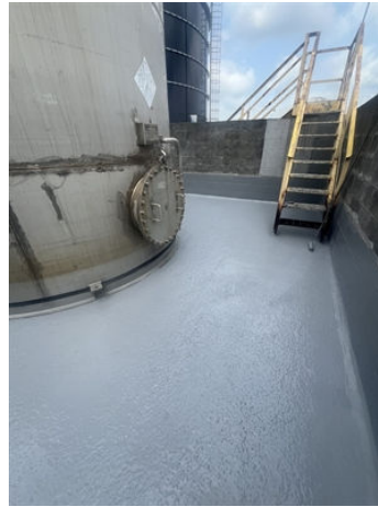
Floor after the second coat
