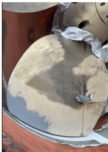
Belzona 1311 applied in areas of cavitation
