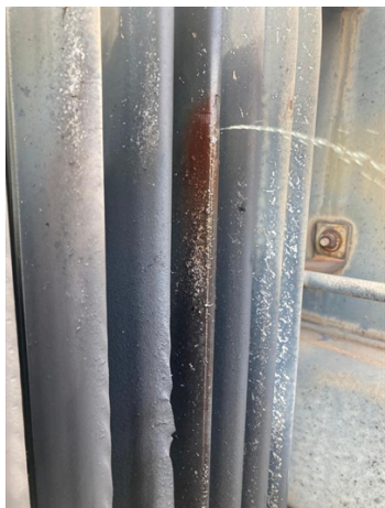
Leaking transformer
