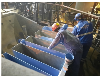
Application of the first layer of Belzona 1341.
