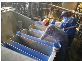
Application of the first layer of Belzona 1341.
