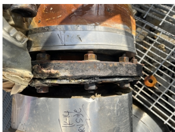
One of the flanges before surface preparation.
