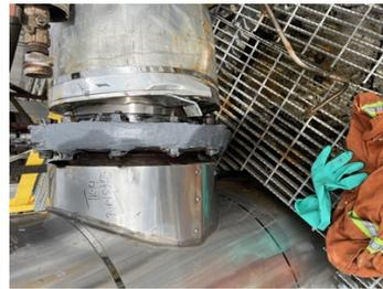
Flange after sealing with Belzona 1212.
