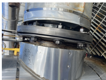
Flange after surface preparation.
