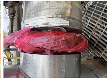
Repair completed with Superwrap II to protect against moisture ingress.
