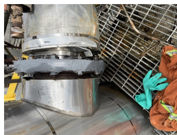
Flange after sealing with Belzona 1212.
