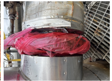
Repair completed with Superwrap II to protect against moisture ingress.
