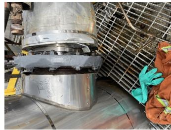
Flange after sealing with Belzona 1212.
