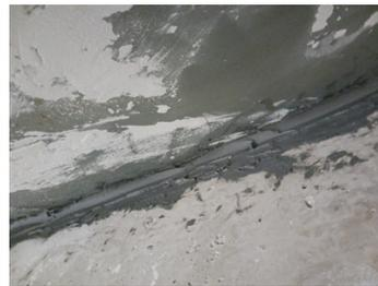
Gap after sealing with Belzona 1111.
