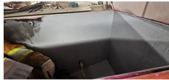
After wrapping top part of tank with superwrap II, the internal is being coated with Belzona 1341.
