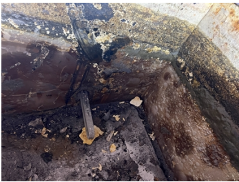
Tank before surface preparation.
