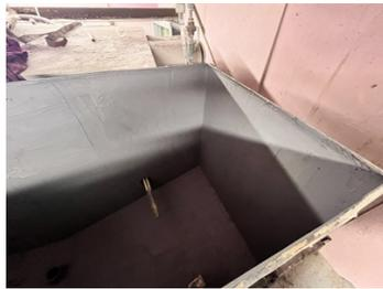
Tank after surface preparation and rebuilding with Belzona 1121.
