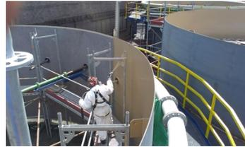
Application of the first layer of Belzona 5811.
