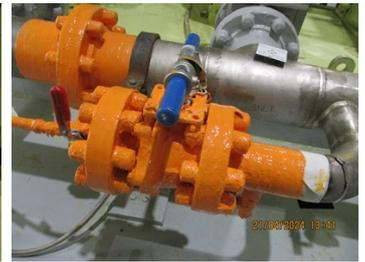
BELZONA 3412 CAN BE APPLIED TO ALL GEOMETRIES AND SEAL THE FLANGE AND FASTENINGS, EASY INSPECTION AND RESEAL.
