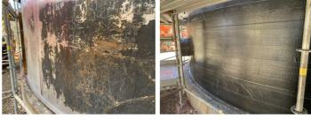
Corrosion under insulation on an ammonium sulphate feed tank
