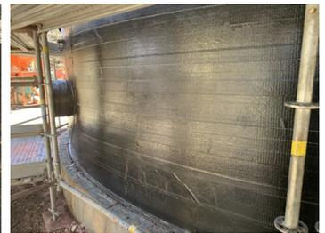
Corrosion under insulation on an ammonium sulphate feed tank
