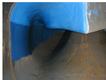
Belzona 1341 application
