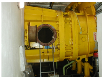
View from the outside
