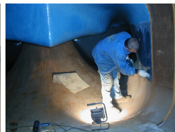
Belzona 1341 application
