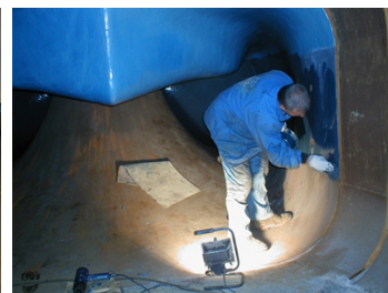
Belzona 1341 application
