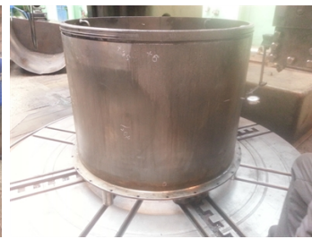
Application of BELZONA 1311
