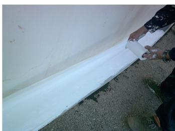
Tank base after the Belzona 3211 application.
