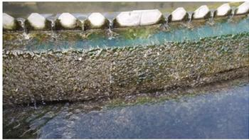
Constant water running over the weirs has caused damage to the concrete
