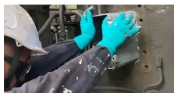
Inserting a piece of the equipment into the repair site.
