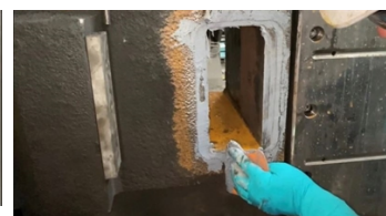
Finished repair with the Belzona products applied.
