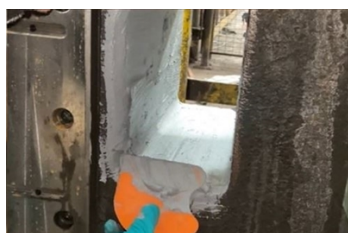
Application of Belzona 1111 to the application site.
