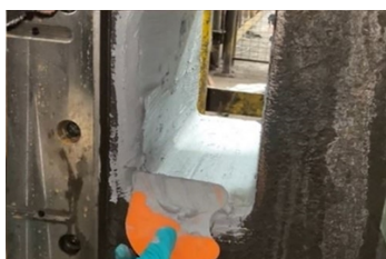
Application of Belzona 1111 to the application site.
