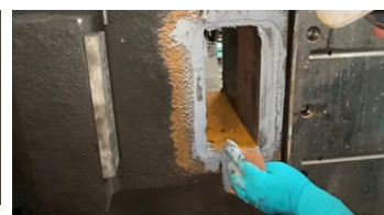
Finished repair with the Belzona products applied.
