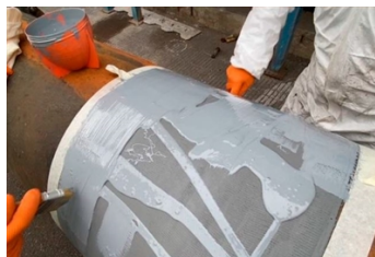
Application of Belzona 5811.
