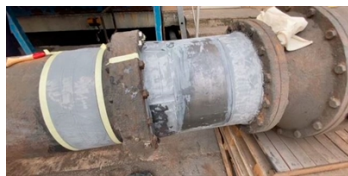
The pipe after being repaired with Belzona 1121.
