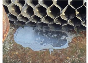
This Belzona 1212 and reinforcement metal is covering about 6" of moderate size pinholes.
