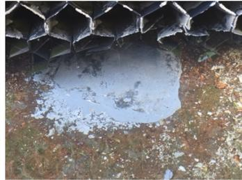
The large hole covered with Belzona 1212 and some reinforcement metal.
