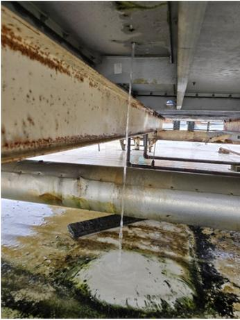
The constant stream of water leaking from the largest hole.
