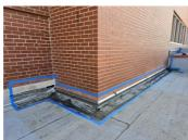
The repair area cleaned, prepped, and taped off.
