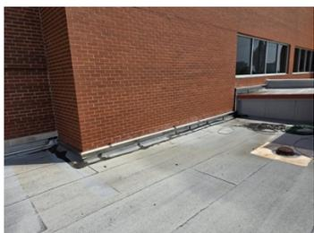
Original condition of the roof showing where other roof repair materials had been applied that failed.
