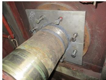
The gasket area former in place with Belzona 1111.
