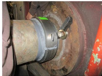
The shaft former in place showing the excess Belzona 1111 squeezing out.
