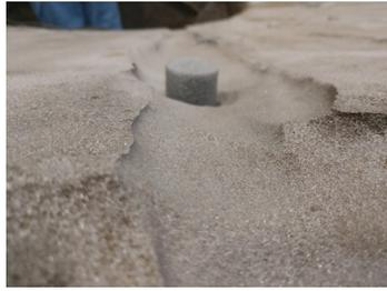
Backer rods inserted into the wear plate mounting holes and showing the target profile height.
