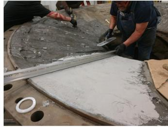
Applying Belzona 4911 Conditioner in the background, and applying Belzona 4111 using a guide to achieve the proper profile.
