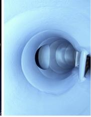
Belzona protective coating from around 2006 was due for a refurbishment
