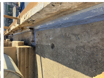
Belzona 3121 Completed
