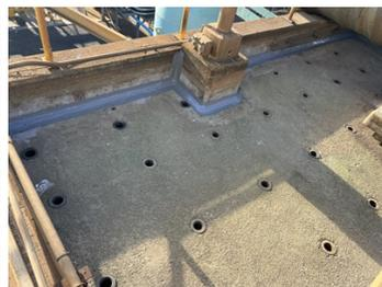
Belzona 3121 Applied with Reinforcement Cloth
