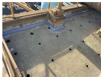
Belzona 3121 Applied with Reinforcement Cloth
