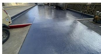
First coat of Belzona 4311 Applied
