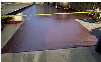
2nd and Final Coat of Belzona 4311 Applied Incorporating Aluminum Oxide for a nonskid finish
