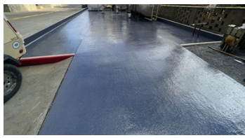
First coat of Belzona 4311 Applied
