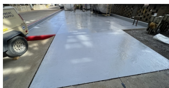
Base Coat Used was Belzona 5811
