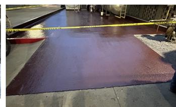
2nd and Final Coat of Belzona 4311 Applied Incorporating Aluminum Oxide for a nonskid finish
