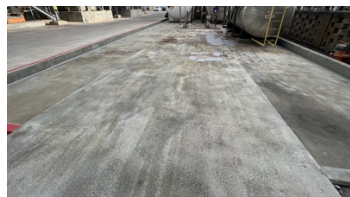
Blasted and Prepared Containment
