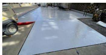
Base Coat Used was Belzona 5811
