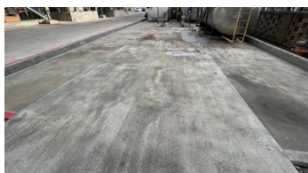
Blasted and Prepared Containment
