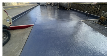
First coat of Belzona 4311 Applied
