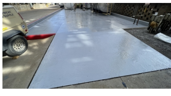
Base Coat Used was Belzona 5811
