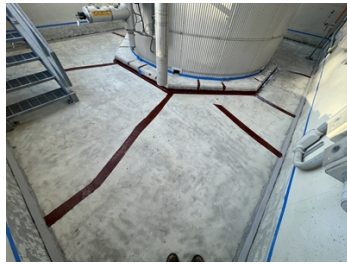
Addressed Cracks and Seams with Belzona 4361 and composite tape
