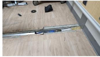
Plate removed and condition of underlying joint
