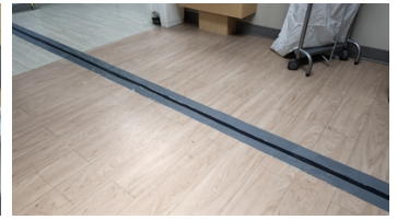
Completely re-engineered and rebuilt smooth ride joint
