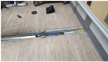
Plate removed and condition of underlying joint
