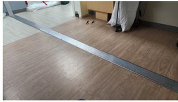
Aluminum cover plate causing bump and trip hazard
