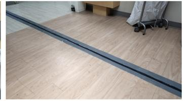
Completely re-engineered and rebuilt smooth ride joint
