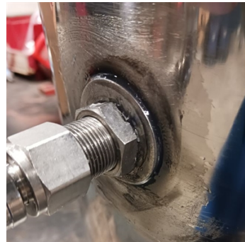
External fitting showing seal of Belzona 2311
