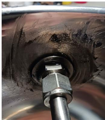
Internal Fitting showing seal of Belzona 2311
