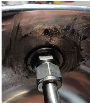
Internal Fitting showing seal of Belzona 2311
