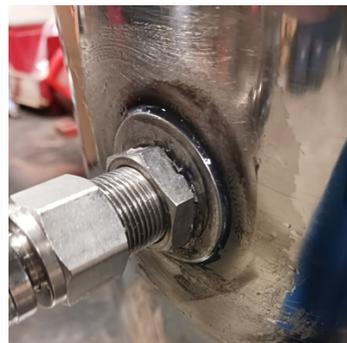
External fitting showing seal of Belzona 2311
