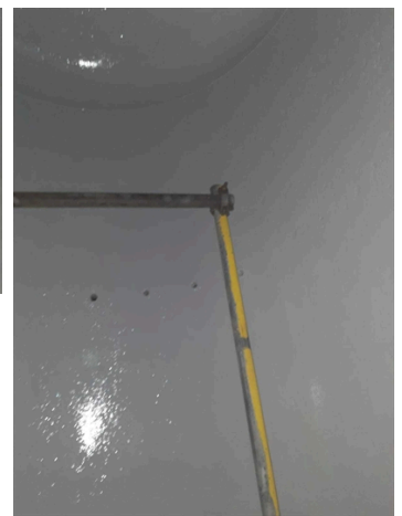
After final coat completed
