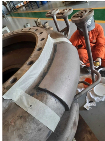
COMPLETED PLATE BONDING USING BELZONA 1311
