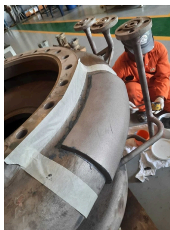
COMPLETED PLATE BONDING USING BELZONA 1311
