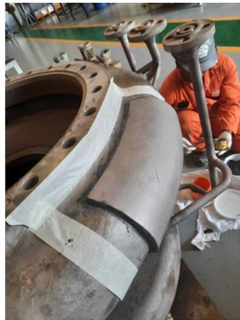
COMPLETED PLATE BONDING USING BELZONA 1311
