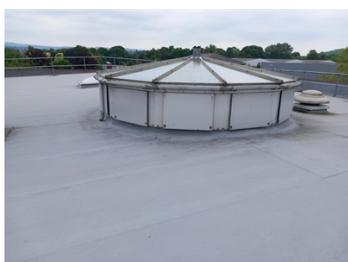
Showing no deterioration to applied Belzona 3131 coating
