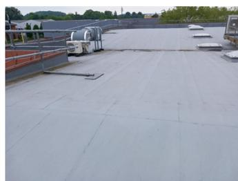
A larger expanse of the main roof where the Belzona 3131 was applied
