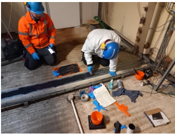
Setting out the works
