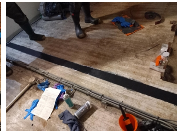
Masking removed showing the completed works
