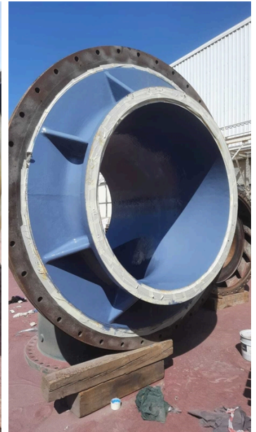
fourth and final coat completed
