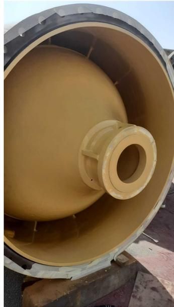
Application of first and second coat was completed and in this is the completed third coat application.
