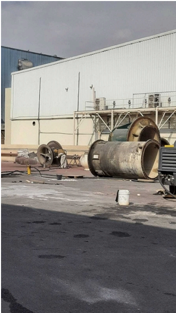
BRP pump status before surface preparation
