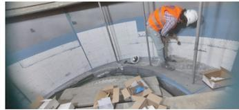
Applying Belzona 9811 Almina Tiles with Belzona 1391T as the adhesive
