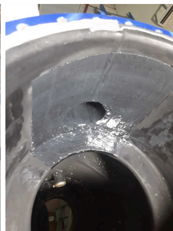
RUBBER LINING REPAIR COMPLETED
