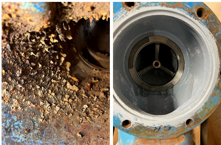
This is a pic of the inside of the backflow preventer before This is a pic of the backflow preventor after
