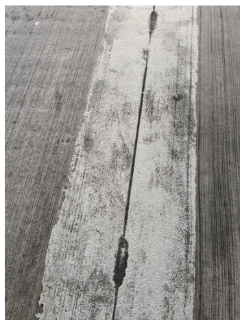
Close-up of the expansion joint. Finished application. needing repair.
