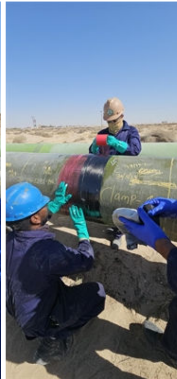
Application of Belzona Superwrap II
