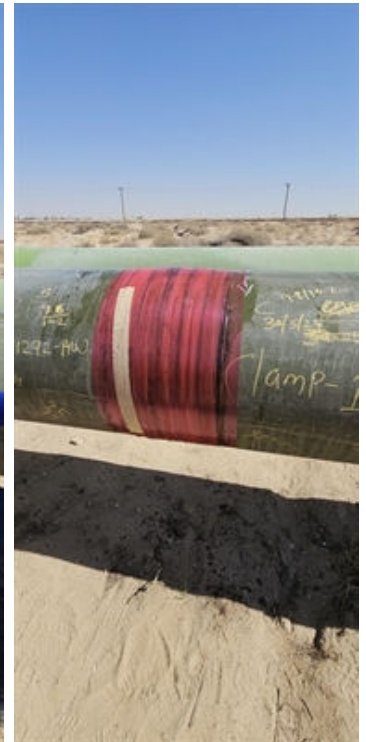
Completed Belzona Superwrap II repair
