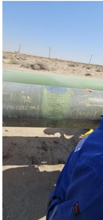
Steel plate bonded using Belzona 1212
