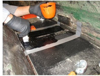
Scrubbing the Belzona 2111 into the application area.
