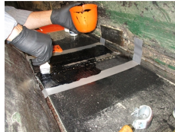
Scrubbing the Belzona 2111 into the application area.
