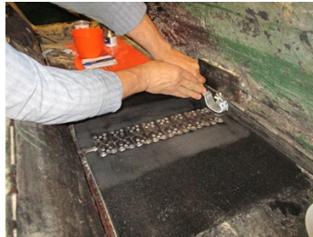
Roughening the surface by hand prior to applying the Belzona 2911 conditioner.
