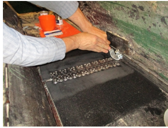
Roughening the surface by hand prior to applying the Belzona 2911 conditioner.
