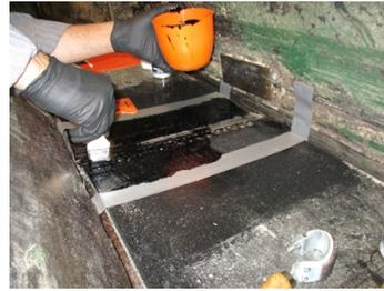
Scrubbing the Belzona 2111 into the application area.
