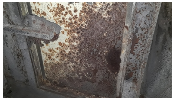
A close up of the general condition of the internal bay's steelwork
