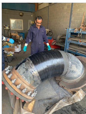
Trial/demo application of Belzona SuperWrap II as per the engineered design.
