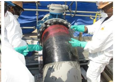
Trial/demo application of Belzona SuperWrap II as per the engineered design.
