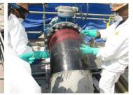
Trial/demo application of Belzona SuperWrap II as per the engineered design. No trace of any leak or peel-off SuperWrap II application for SuperWrap II application by after the completed hydrotest. 24-inch elbow of 3.6 m length. distributor
