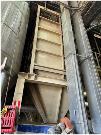
Hopper was approximately 2 storeys high.
