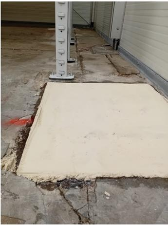
Uneven floor area made good using Belzona 4111 MagmaQuartz to support main racking stanchions
