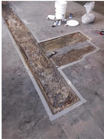
Damaged area prepared and conditioned with Belzona 4911 ready to accept Belzona 4131 MagmaScreed
