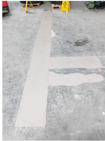
Damaged area fully repaired, screeded and feather edged with Belzona 4131 MagmaScreed to provide flat safe running surface for fork lift trucks and handling machinery
