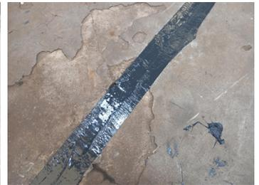
One of 5 expansion joints raked out, cleaned, conditioned with Belzona 2911 Conditioner and finished with Belzona 2211 Hi-Build elastomer
