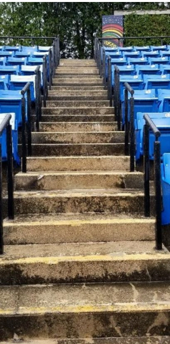
State of the steps before renovation project
